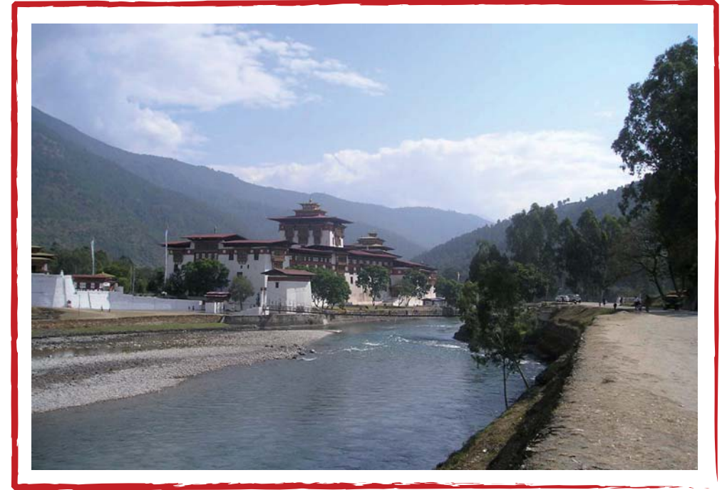
Punakha Dzong with steel suspension bridge, ungainly provisional solution 1958-2007
