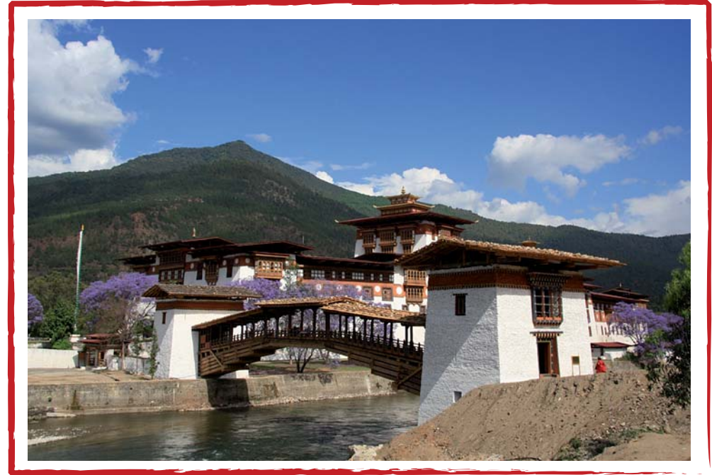
New bridge seen from Punakha village, 10. May 2008
